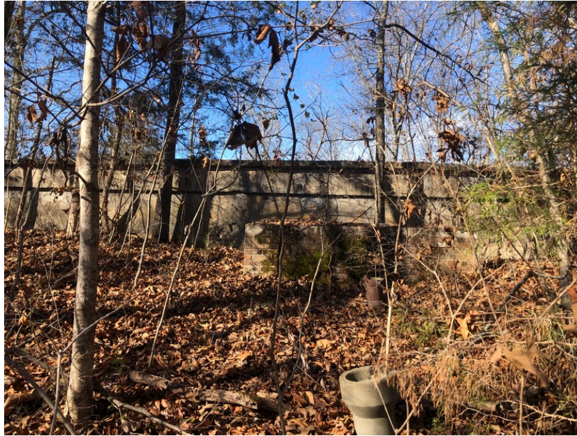
Photograph 13: View of the Clinton Reservoir located on the north adjoining property.
